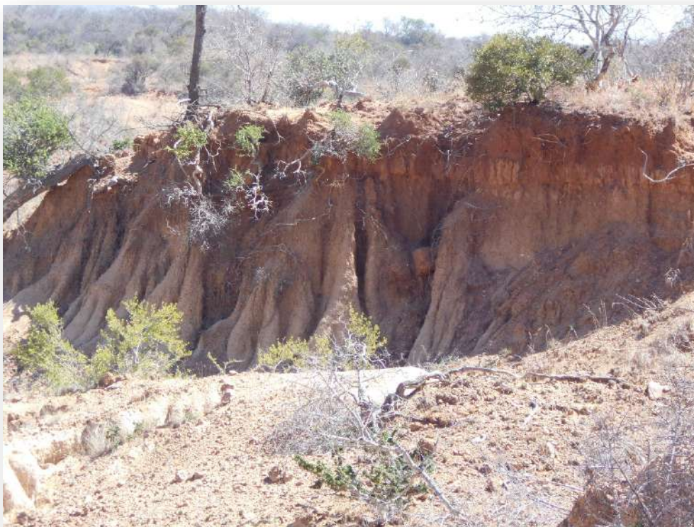
Plate 3.2 Erosion typically associated with the non-perennial drainages on the Thorny River project
